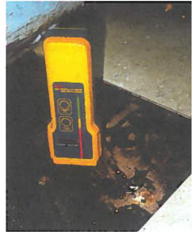
Photo 9: Moisture meter measuring moisture content of plywood subfloor
